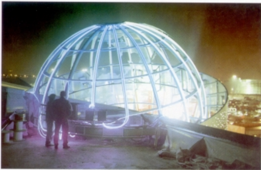
Fig. 2: A rear view from the theater roof shows the brightness of SuperVision's 1/4-in. FO cables after dark.
