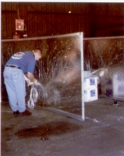
Fig. 4: Dan Myers of Fiber Productions installs thousands of tiny FO strands through small holes in sections of the equatorial aluminum band.
